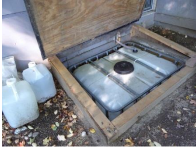
Outdoor storage tank (urine)
